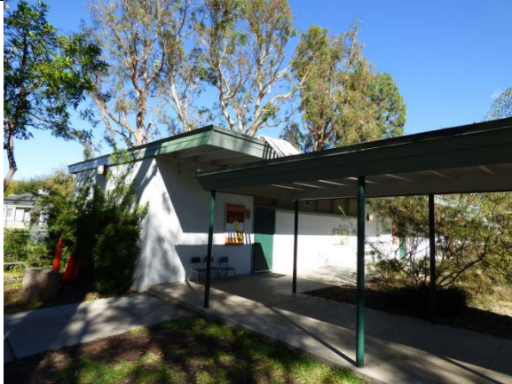
Classroom Building 10/G, South and West Elevation, View Southeast
