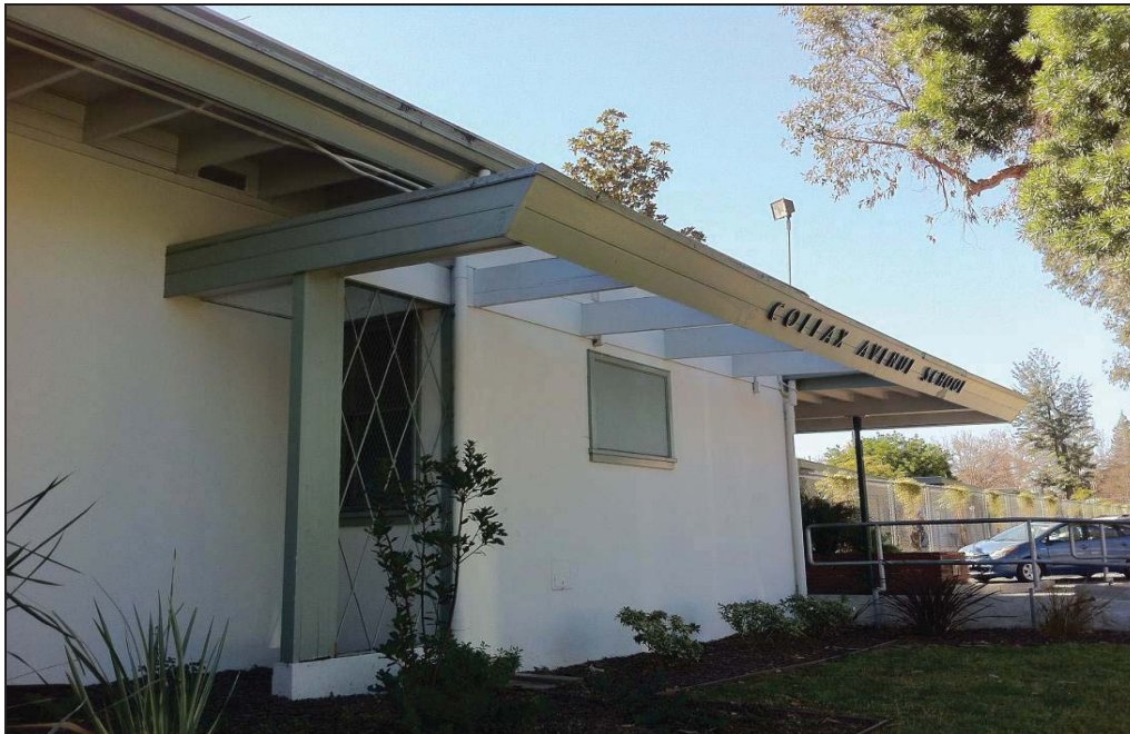
Colfax Avenue Elementary School, detail, Administration Building. Eaves extend to form an open grid around the entrance wing. Northeast perspective. Source: Sapphos Environmental, Inc., 21 January 2014.
