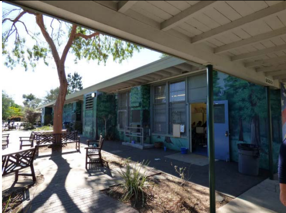
Classroom Building 4/C, East Elevation, View Southwest
