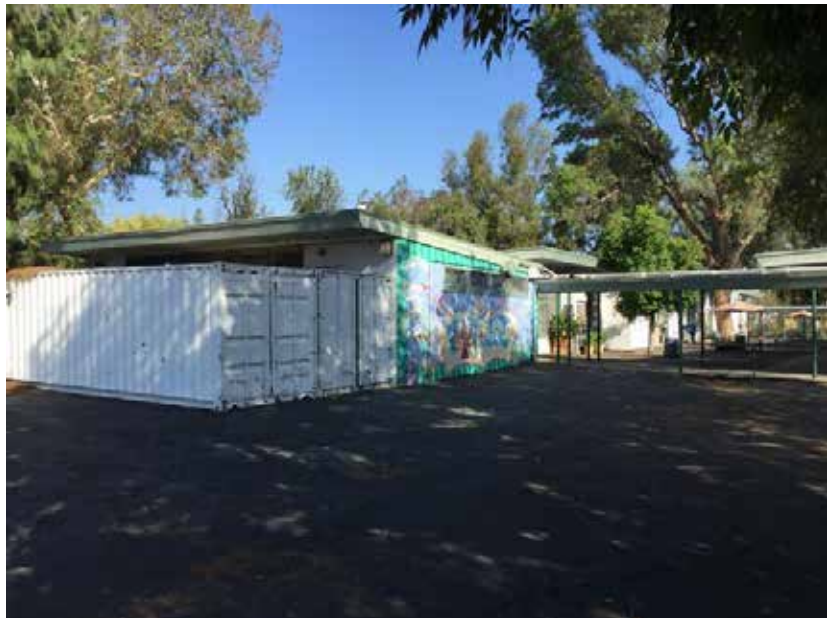
Photo 8: Northwest portion of the Site, viewing the intermodal container storing non-hazardous materials, looking northwest.
