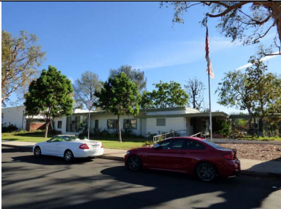
Administration Building 1/A, North Elevation, View South
