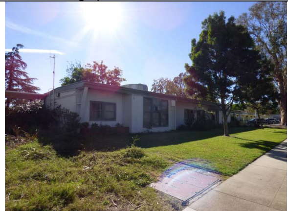
Administration Building 1/A, North Elevation, View Southwest
