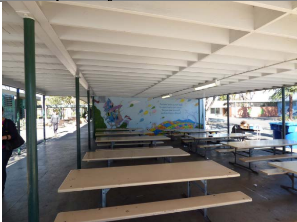
Library Building 3, Under Lunch Cover, South Elevation, View North
