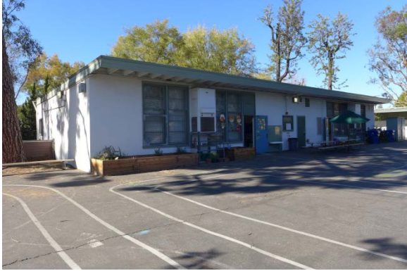
Kindergarten Classroom Building 11/H, South and East Elevations, View Northwest
