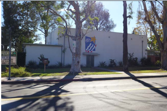
Multi-Purpose Building 2, North Elevation, View South
