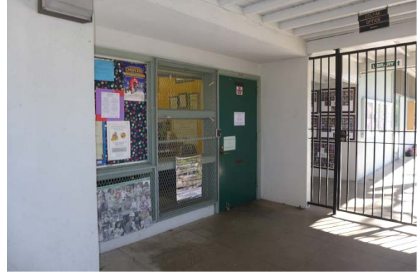
Administration Building 1/A, Side Entrance on West Elevation, View East
