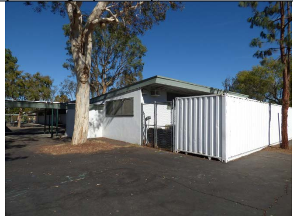
Sanitary Building 9/J, West and Rear (South) Elevations, View Northeast, Note non-contributing storage units
