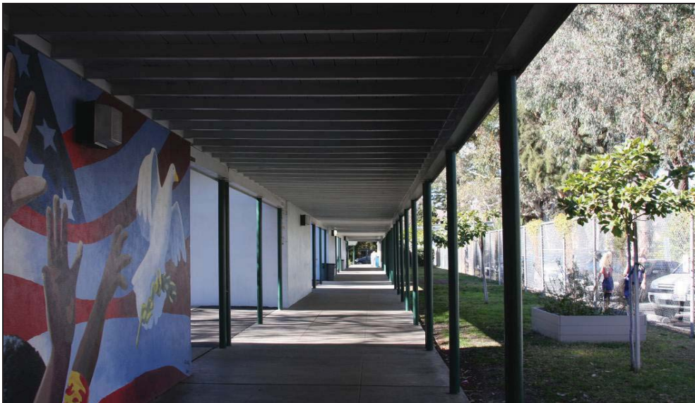
Colfax Avenue Elementary School, arcades connect all classrooms along the north and south expanses of campus. East perspective. Source: Sapphos Environmental, Inc., 21 January 2014.
