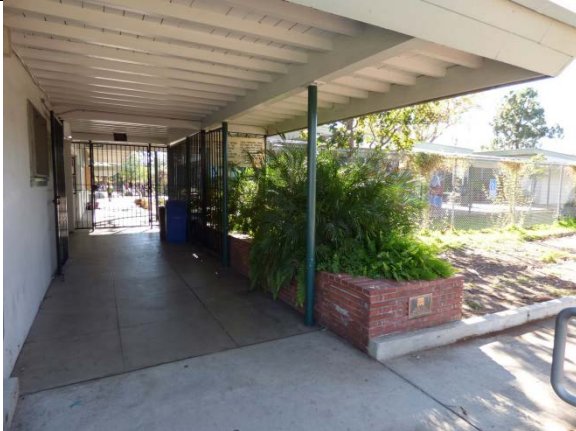
Administration Building 1/A, Entrance, View South, Note Brick Planter and Trellis at South-end
