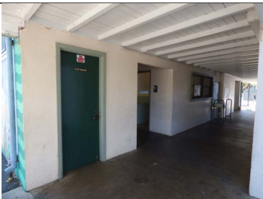
Sanitary Building 9/J, North Elevation, View Southwest
