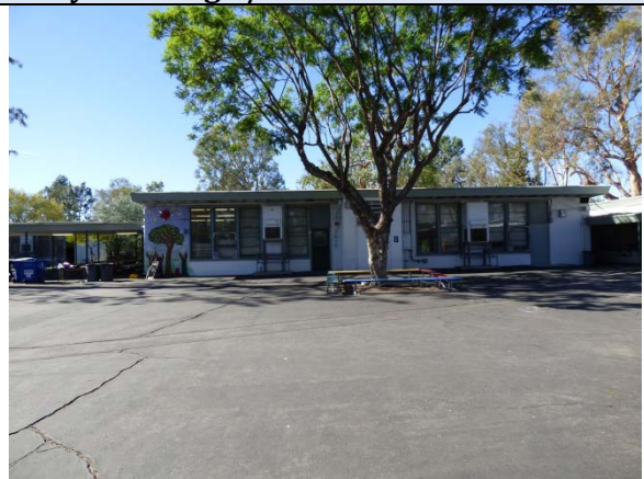
Library Building 3, East Elevation, View West
