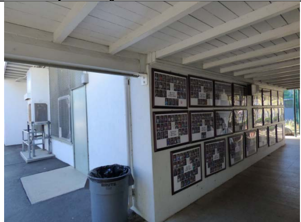
Library Building 3, Under Covered Walkway, North Elevation, View Southwest
