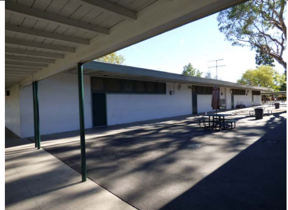
Classroom Building 5/D, West Elevation, View Southeast
