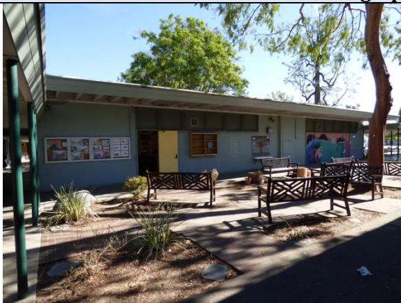
Library Building 3, West Elevation, View East
