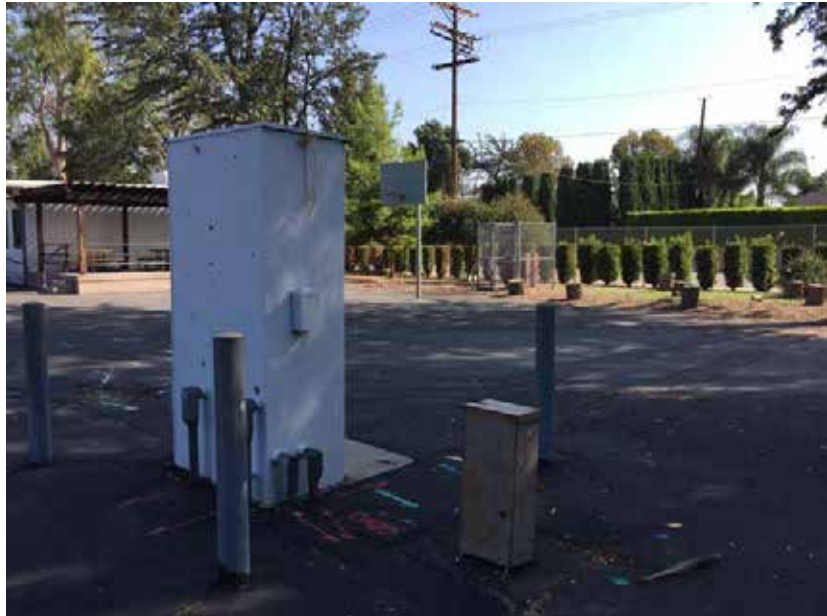
Photo 12: From left to right, electrical box and electrical sprinkler box, and electrical transformer further in the background, looking northeast.
