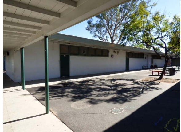
Classroom Building 6/E, West Elevation, View Southeast
