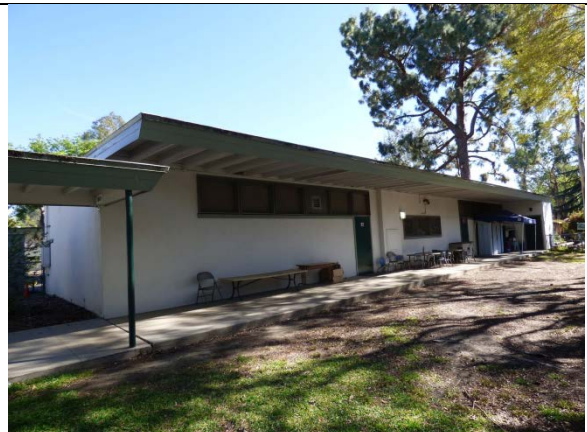
Kindergarten Classroom Building 11/H, North and West Elevations, View Southeast
