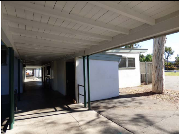
Sanitary Building 9/J, West Elevation, View East
