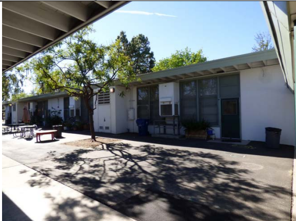
Classroom Building 7/F, East Elevation, View Southwest
