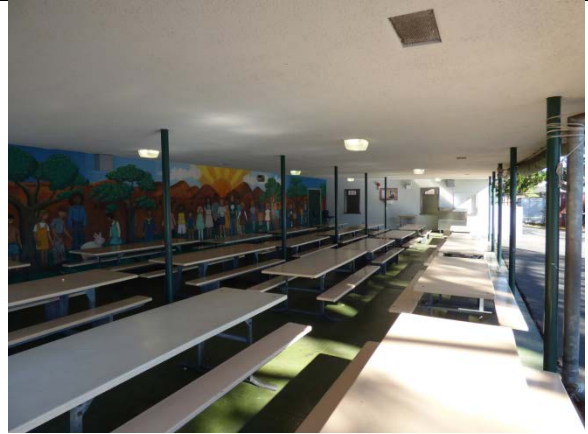
Multi-Purpose Building 2, View Northwest under Lunch Cover
