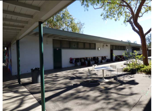
Classroom Building 4/C, West Elevation, View Southeast
