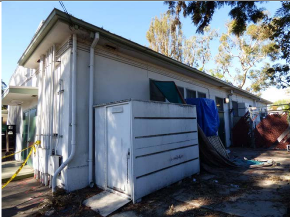
Multi-Purpose Building 2, East Elevation of Lunch Room, View Northwest
