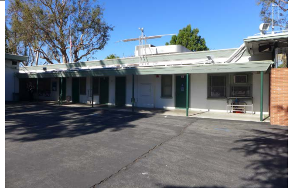
Administration Building 1/A, South Elevation, View North
