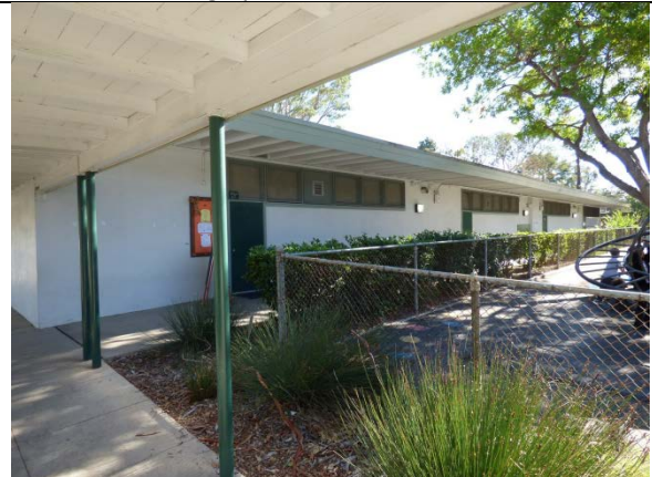
Classroom Building 7/F, West Elevation, View Southeast
