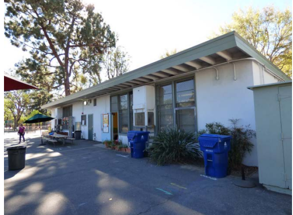
Kindergarten Classroom Building 11/H, East Elevation, View Southwest
