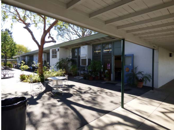
Classroom Building 5/D, East Elevation, View Southwest
