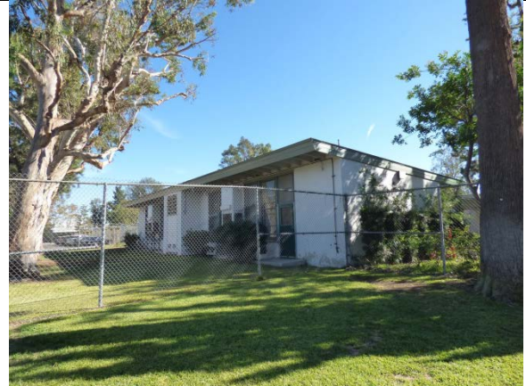
Classroom Building 10/G, West and North Elevation, View Southeast
