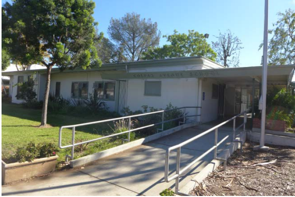
Administration Building 1/A, North Elevation, View South
