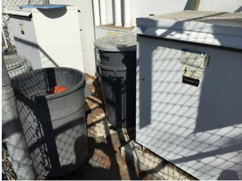
Photo 13: Transformer no. 1 and 2, located in the mid portion of the Site near classroom 20, looking northeast.
