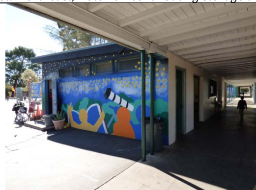
Sanitary Building 8/K, East Elevation, View West
