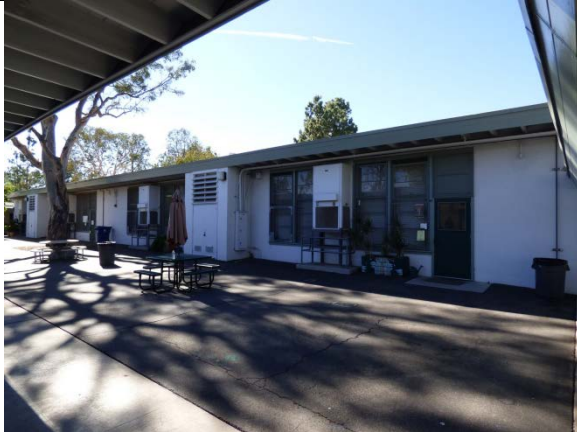
Classroom Building 6/E, East Elevation, View Southwest
