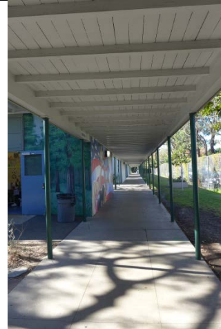
Covered Walkway/Arcade Connecting the North Elevations of Buildings 3 to 7, View West
