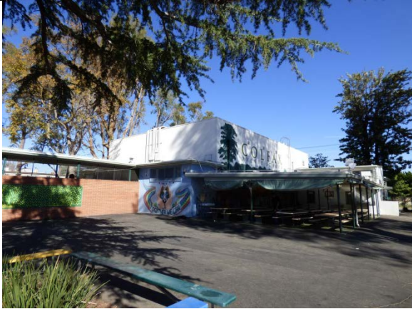
Multi-Purpose Building 2, West and South Elevation, View Northeast
